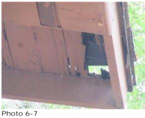
7 - Rot was found in one or more areas on fascia boards. A qualified contractor should evaluate and make repairs as necessary, replacing all rotten wood.
